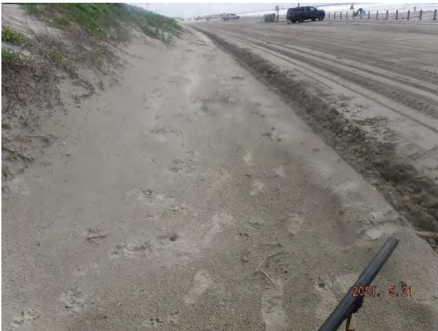
Picture 81: UD11JLM Bearing: Northeast Date: 5/21/2021
