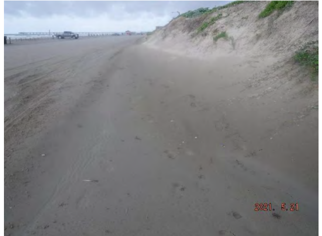
Picture 74: UD10JLM Bearing: West Date: 5/21/2021
