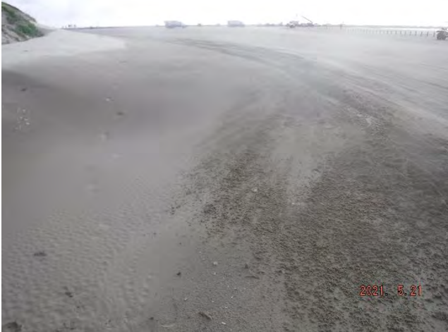
Picture 73: UD10JLM Bearing: Northeast Date: 5/21/2021
