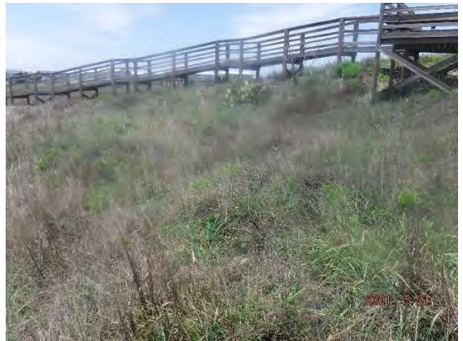
Picture 64: UD09JLM Bearing: North Date: 5/21/2021
